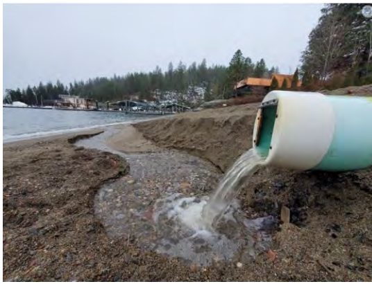
Figure 7. Uncontrolled stormwater outflow causing beach erosion.
